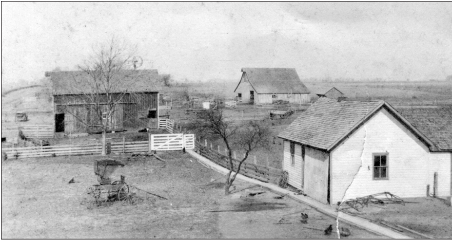
The barns on the J.W. Schwerer farm
