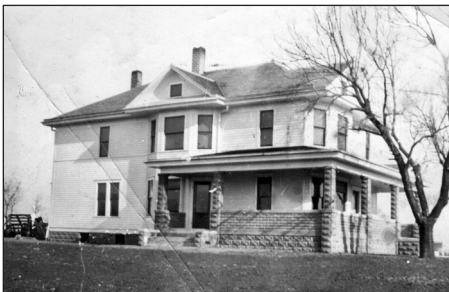
The house that J.W. Schwerer built in 1916
